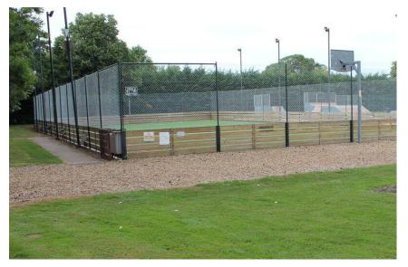
The surface is half filled sand with 13 mm pile.
